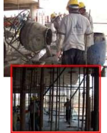
**Fig 15. : Micro concreting in progress**
