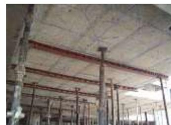
**Fig.9. : Truss Supports to beam**
