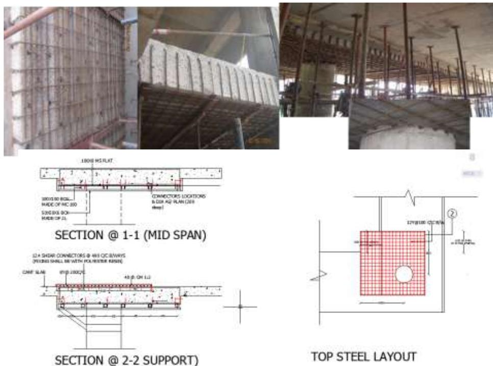
Fig 11 : Reinforcement Details & after fabrication and anchoring
