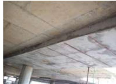
**Fig. 16 : Beam after de-shuttering**
