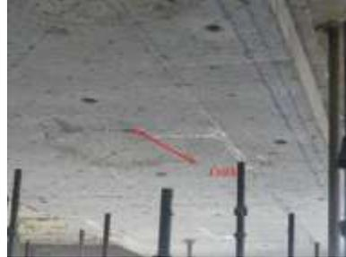
**Fig 4A : Crack in the beam**
